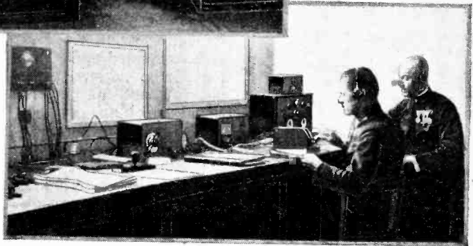
SHORT WAVES FOR THE POLICE. The Hungarian police force has established a wireless organization which includes a number of low power transmitters and more than 230 receivers. The upper picture shows the 800-watt transmitter at Budapest. Below is a typical receiving room.
